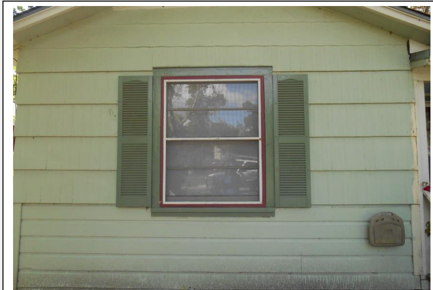
Close-up of one of the windows to be replaced
