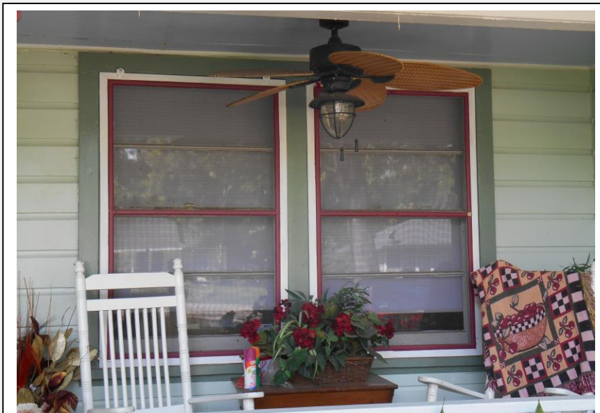
Close-up of the windows on the porch to be replaced
