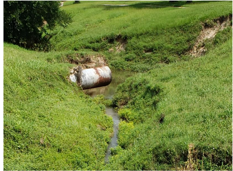
Mag. Creek/Summer Pl Outfall #2 in 2019
