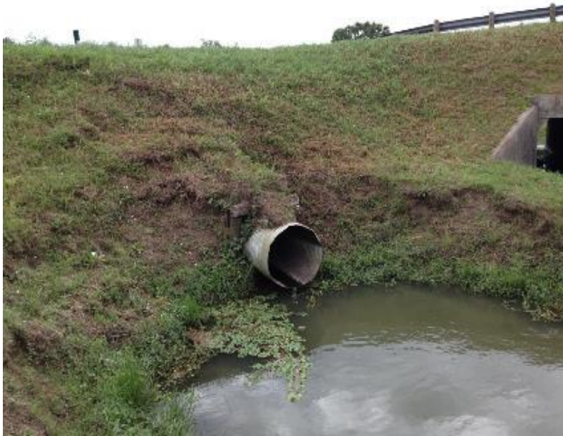
Mag. Creek/Summer Pl Outfall #1 in 2014
