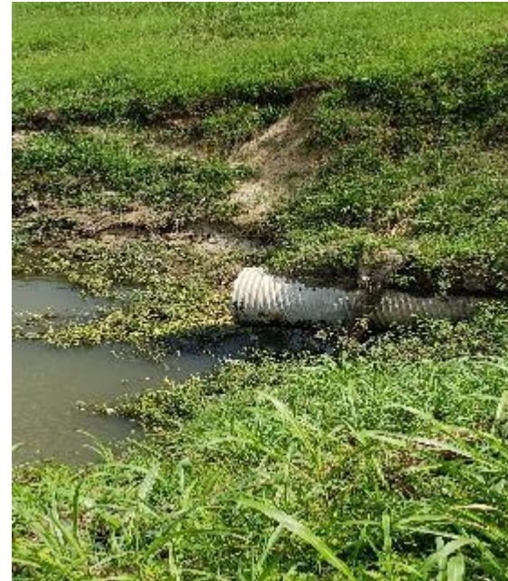
Mag. Creek/Summer Pl Outfall #1 in 2019
