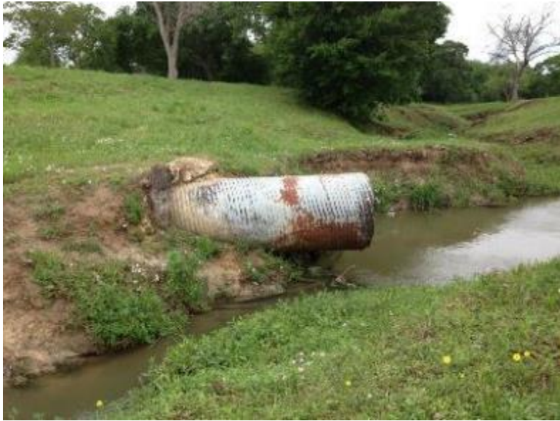
Mag. Creek/Summer Pl Outfall #2 in 2014
